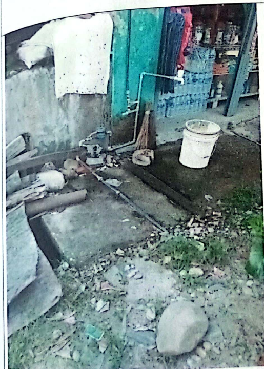
Figure 0.3: Drinking Water Supply Pipeline in the Road Alignment
